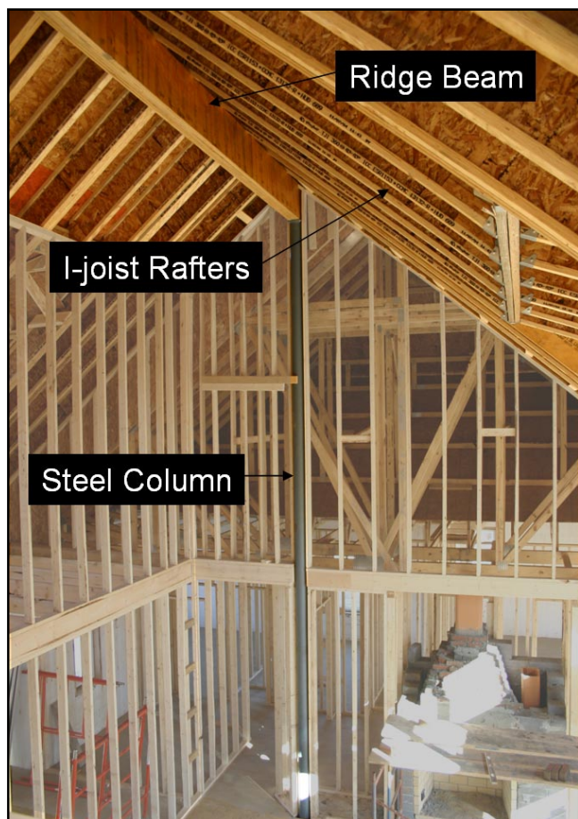
Figure 8 I-Joists Used as Roof Rafters
