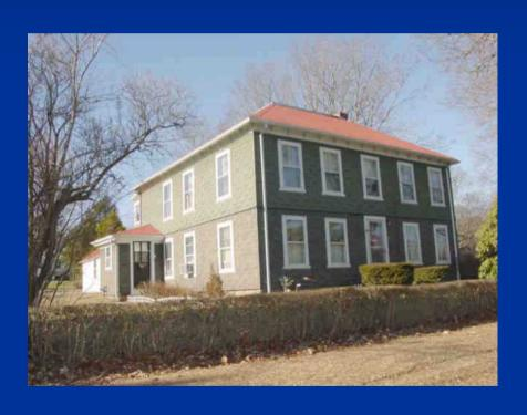
Asphalt or "Gasoline" siding
