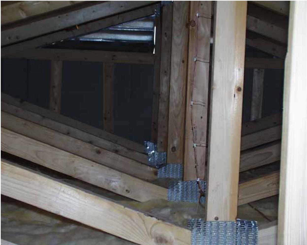
Figure 11. Photograph showing trusses supporting the roof structure with thermocouple array visible in front of second vertical wood member.
