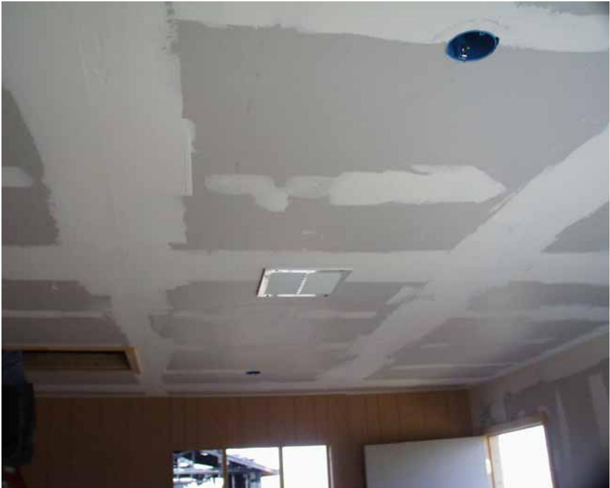
Figure 6. Photograph showing “living room” ceiling with ceiling louvers, electrical boxes, and attic access.
